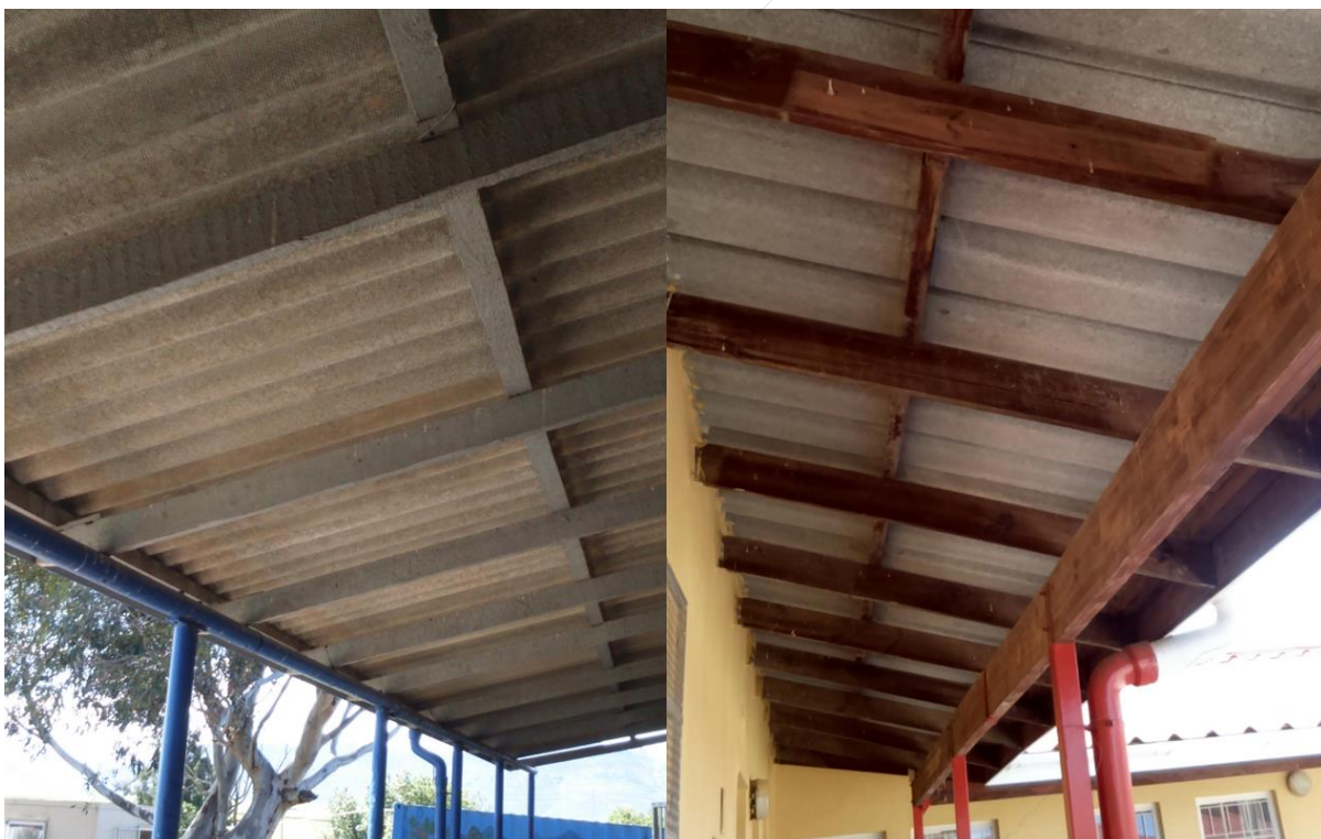
Schools on Private Land: These rural schools have asbestos roofing, which is a health risk for learners and educators. Both are located on private land; the WCED has said that no schools built on private land will receive infrastructure upgrades under the Norms and Standards for School Infrastructure.
