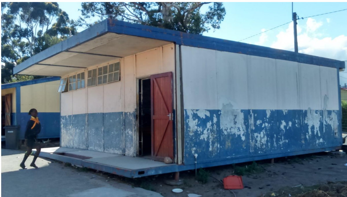
A Container School: More than half of schools included inappropriate structures, some of which were container classes. Many of these installed decades ago and have never been upgraded into proper classrooms. These temporary structures are designed to be exactly that and many begin to fall apart after a few years.
