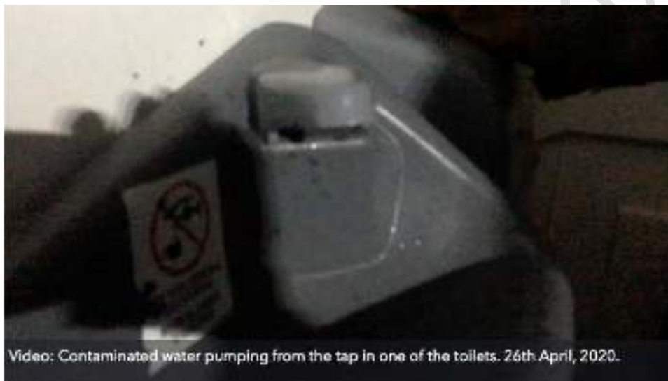
Figure 76: Contaminated water pumping from the tap in one of the toilets, 26 April 2020 (Source: Reverend Annie Kirke)
