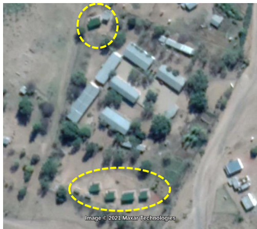
Above: June 2017, five small structures with green roofs have been built to the north and south of the school since June 2016. The research team could not access this site to verify completion. Given the size of these structures and their positions relatively far away from the other classrooms, these are likely toilets rather than the classroom referred to in the SLP. Maps data: Google © 2021 Maxar Technologies
