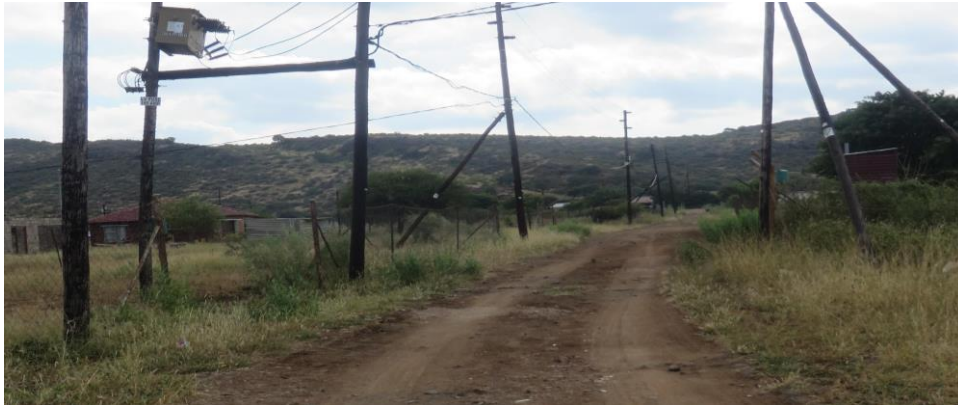
Above: The poor condition of the road at Manyaka village.
