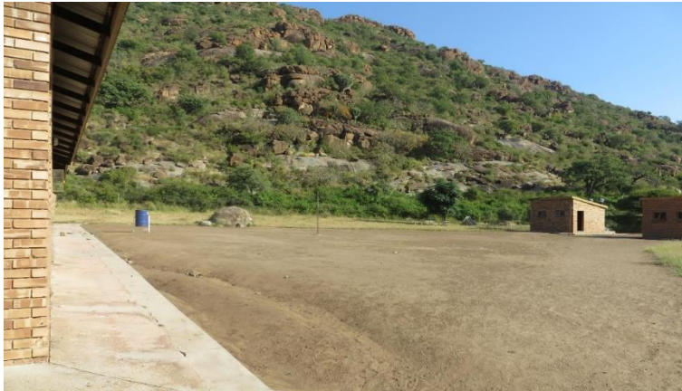
Above: Proposed site for toilets at Maboragane School, which are yet unbuilt. The two buildings on the right house the eight toilets currently serving the school's 175 students and 6 staff members.
